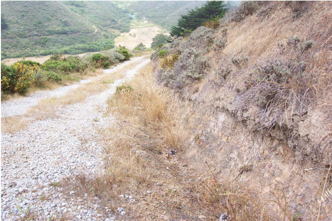
Figure 103: Large gravels spread onto the nearly impervious surface of the road. Over time the gravels will aerate the soils making the road more permeable to moisture.
