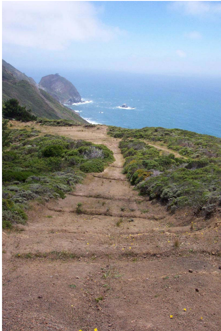
Figure 101: Existing and apparently effective sediment control measures implemented in Pedro Point II subwatershed.
