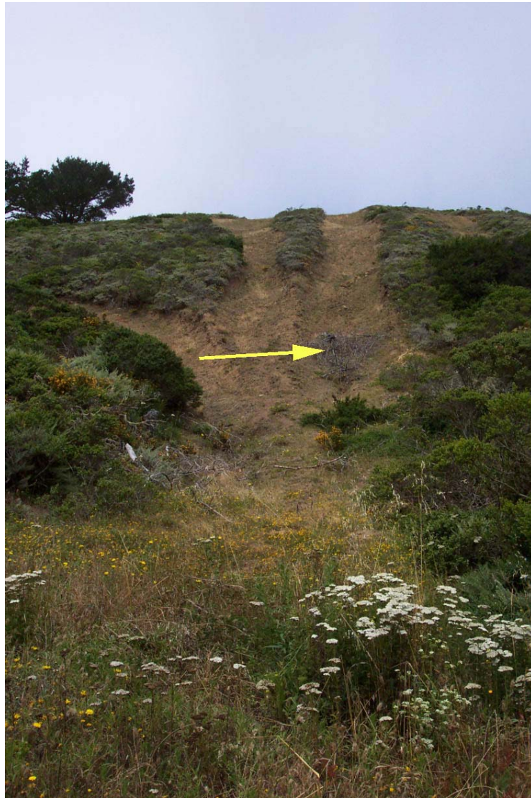
Figure 102: Tree and shrub cuttings (at arrow) placed along trail in an area with deep incision to reduce erosion and promote vegetation growth.
