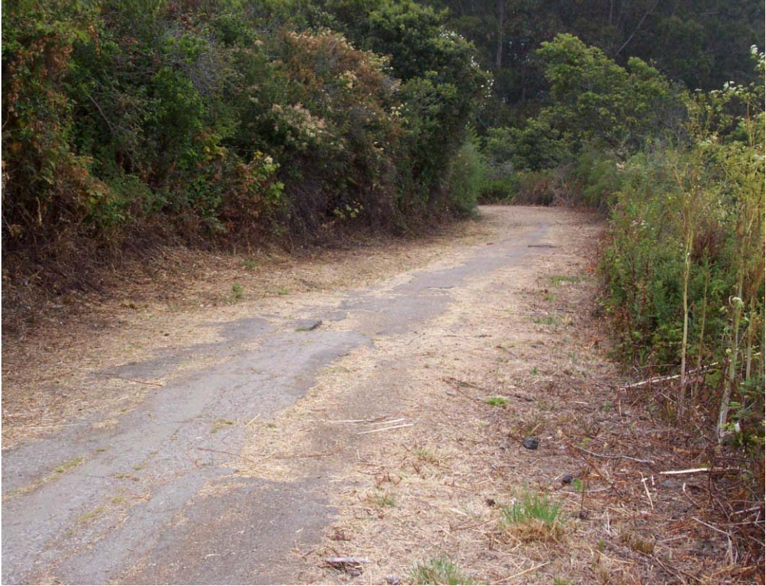
Figure 106: The partially paved surface of the Coastside Boulevard.
