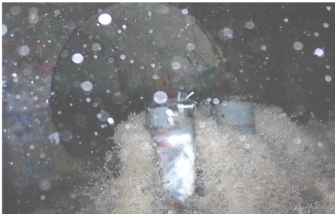
Photo 8. North Fork Culvert flows During the February 11, 2000 Storm
