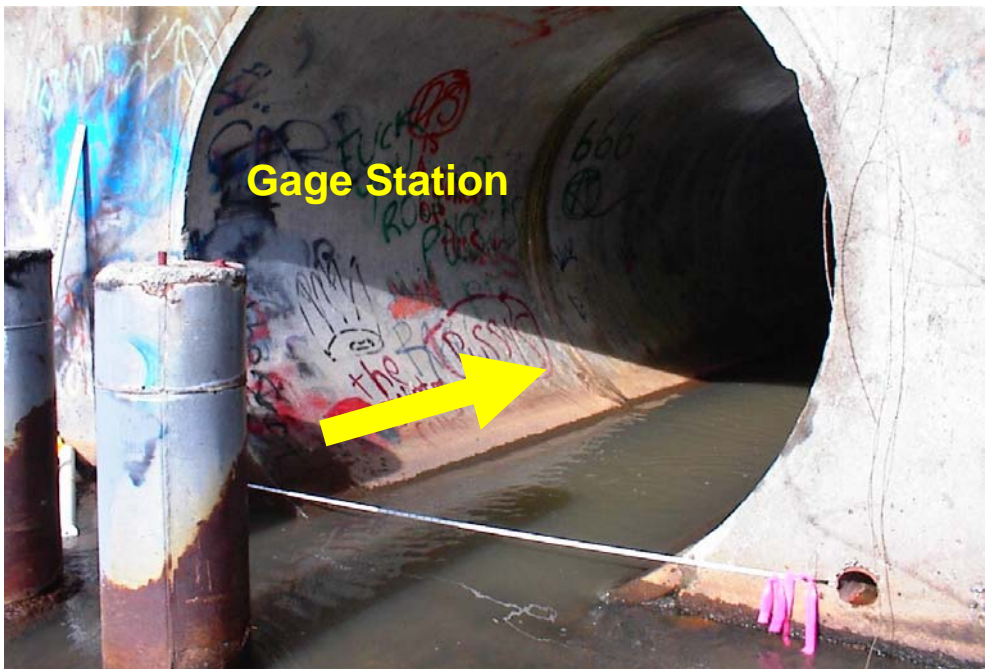
Photo 6. North Fork Culvert
