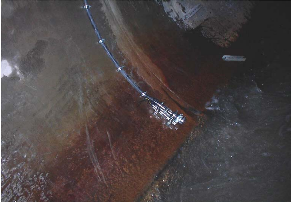
Photo 5. North Fork Gage Station Inside Culvert
